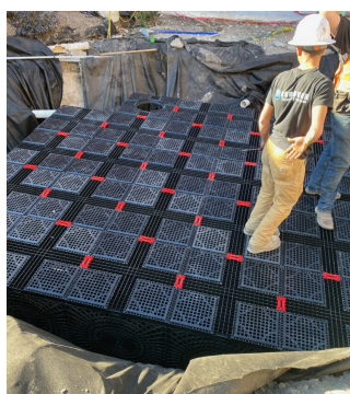
Installation of an Aquabox underground stormwater storage tank.
